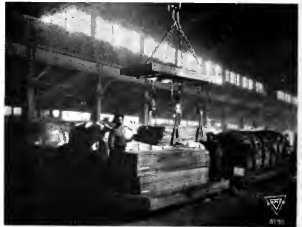
LOADING SHEETS FOR ANNEALING
